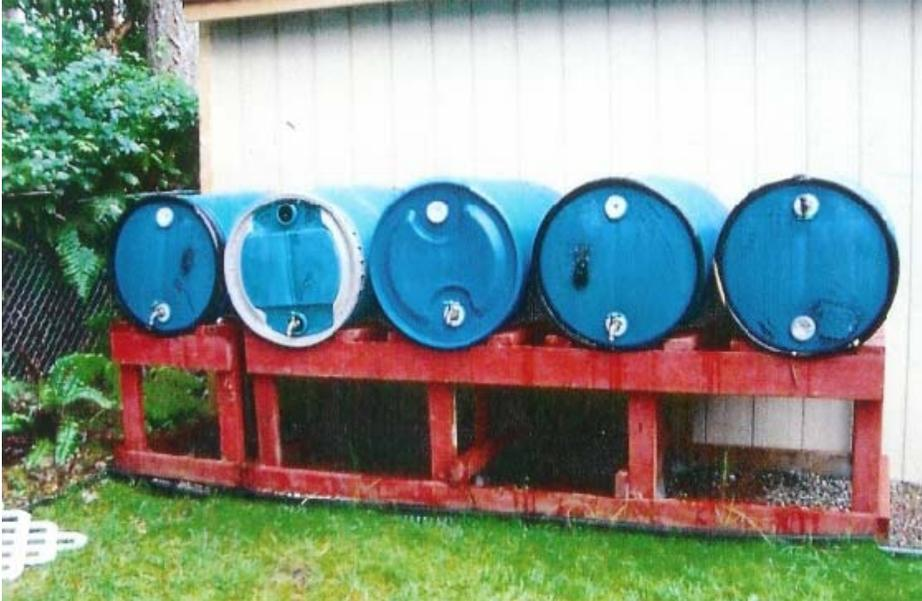
Each of his barrels has a metal spigot on it. The lid for the blue barrels just has a normal garden hose thread in them so you can either put a plastic spigot or a metal spigot in it. Because he used a metal spigot it also has a garden hose thread on the spout end. That way he can just hook a garden hose on it and drain the water out on to the lawn.
