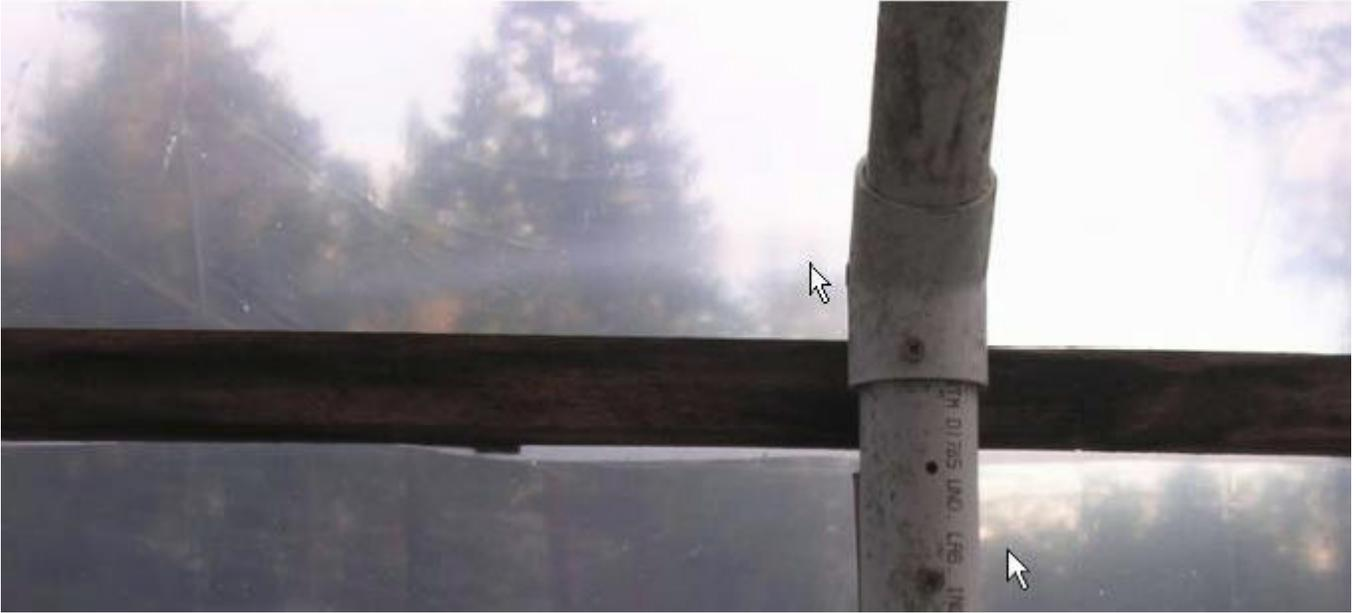
So I have wood at the top and the bottom and all around the ends to hook the plastic too. I put the screws from the PCV pipe side into the wood so the wood would not split from the screws.
