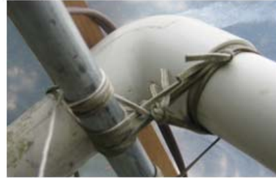
Roof to roof PCV pipe 90 degree angle
